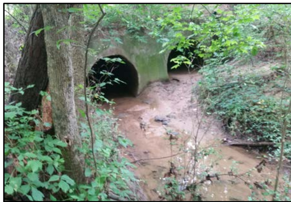
Picture 4-6: Summerfield Crossing – Existing RCPs
