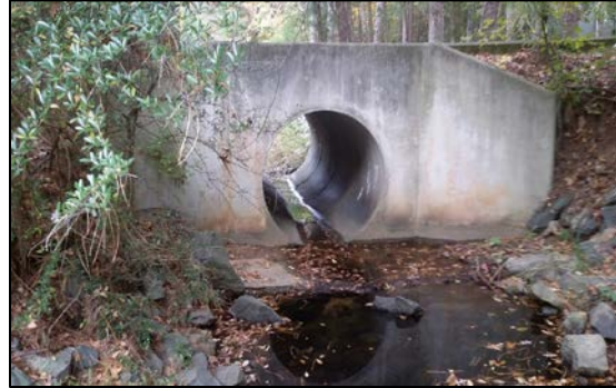
Picture 6-3: Booker 1 looking upstream– Perched Culvert
